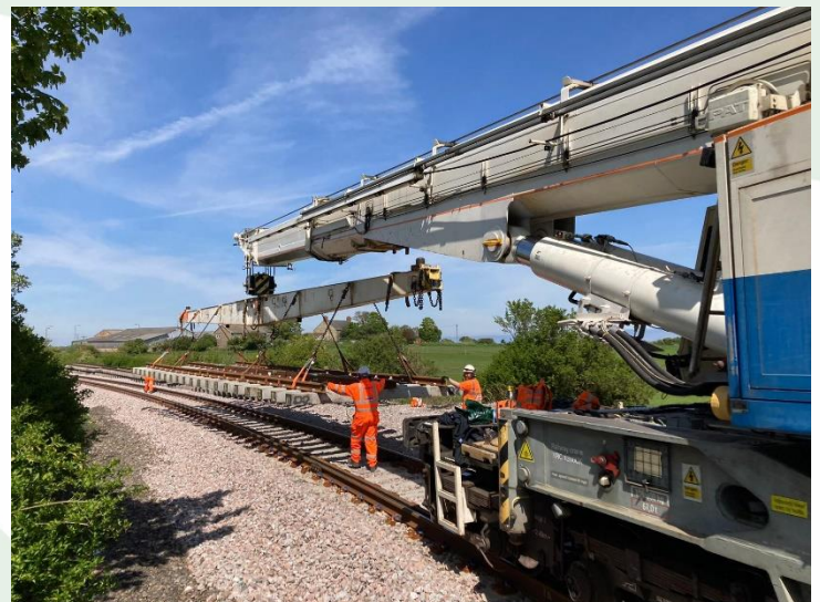
Track upgrade works on the Northumberland Line
