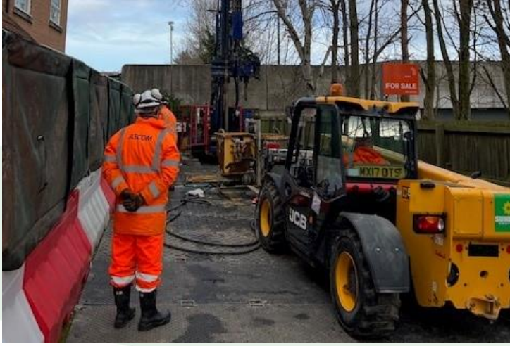
Works in action at Northumberland Park
