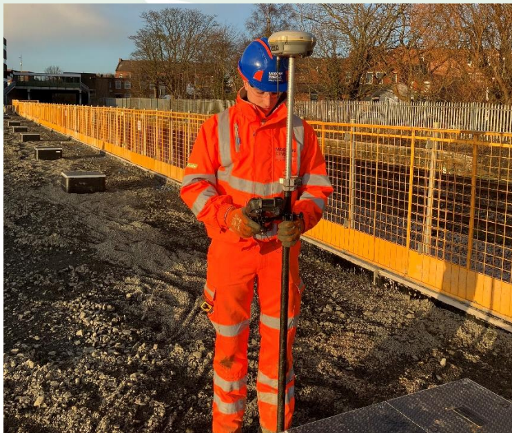
Josh on site at Ashington Station
